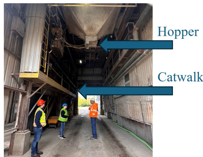
Figure 2: Typical feed truck loading station with a catwalk
